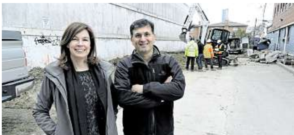
St. Clare's operations manager Andrea Adams, left, and physical assets manager Mohammad Anvari pose at 25 Leonard Ave., where excavation has begun for a three-storey building that will provide purpose-built rentals for homeless people.
