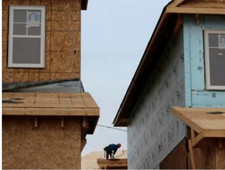
Under construction - File photo
