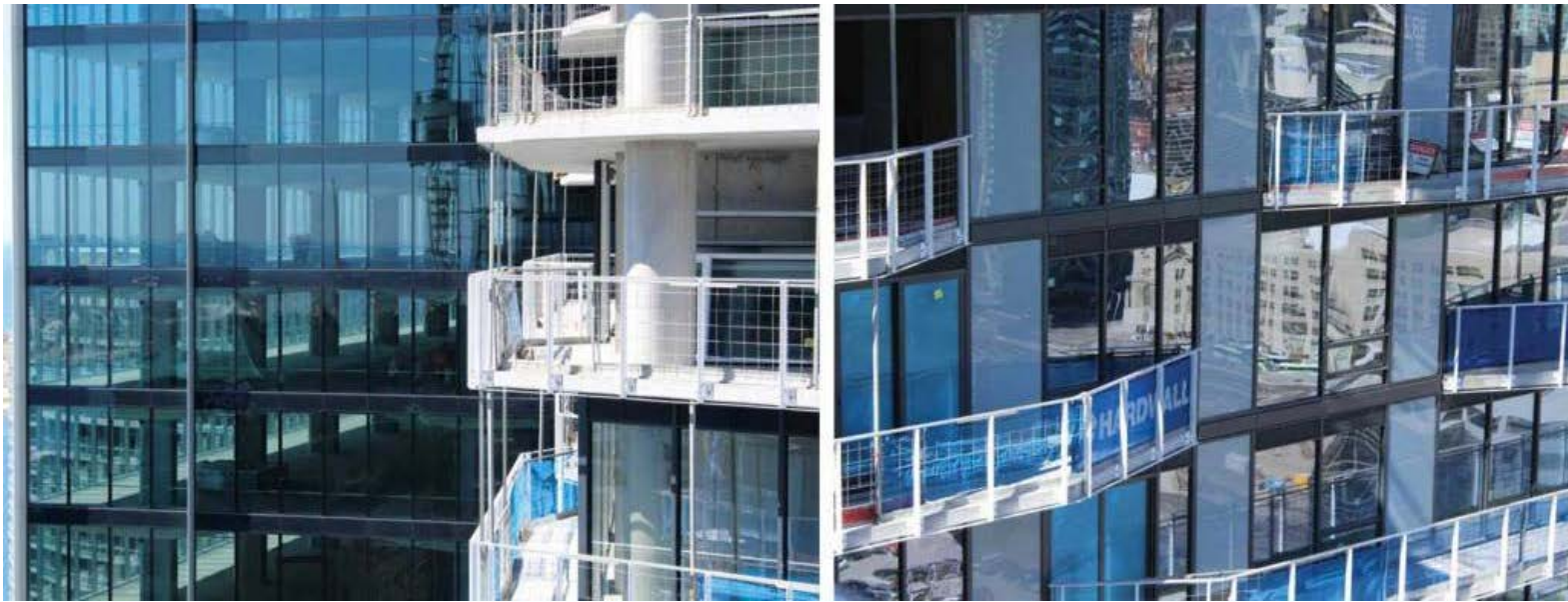
[4] Figure 2: A quick visual comparison of a curtain wall (left) and window wall (right).
