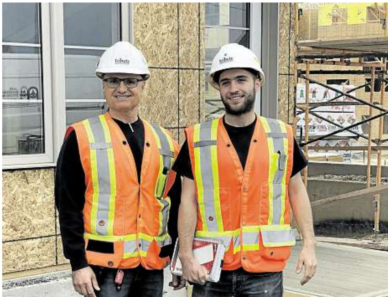
21-year-old Thomas McHardy (right) is one of the youngest employees to come out of the construction management program at George Brown College. Seen here with Frank McPhee, Tribute, v-p of contracts.
