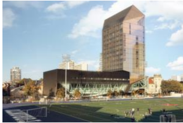
The University of Toronto's proposed 14-storey mass timber and concrete hybrid building.
