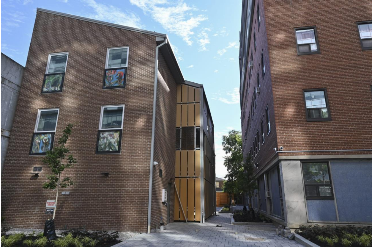
The new affordable rental units at 25 Leonard Avenue.
